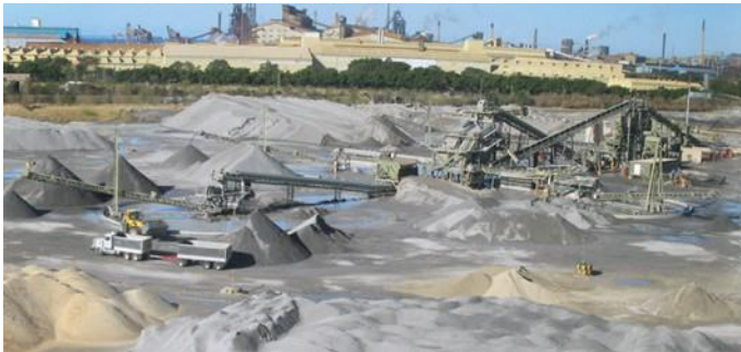
Slag Aggregates Preparation Plant
